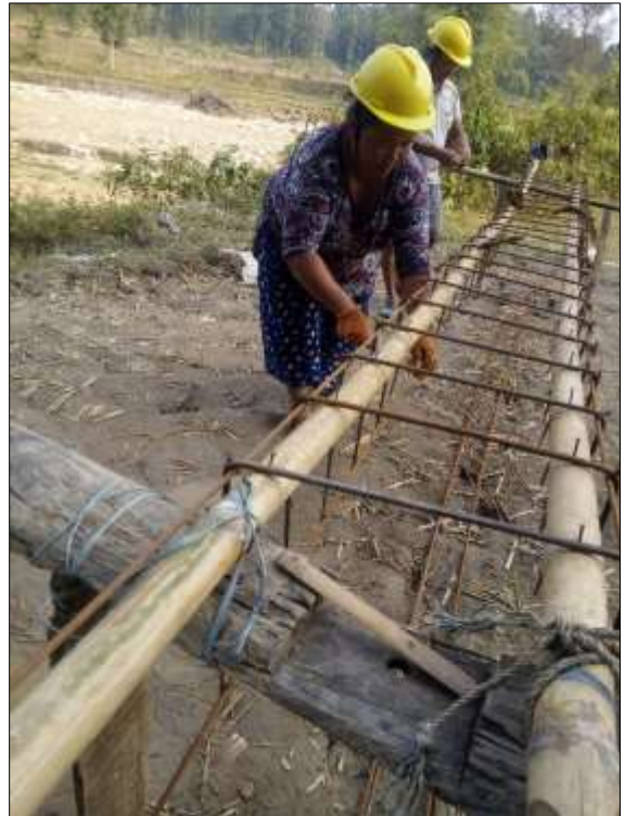
Ms. Rewati Rai binding the reinforcement bar in Bahuni Irrigation Scheme
