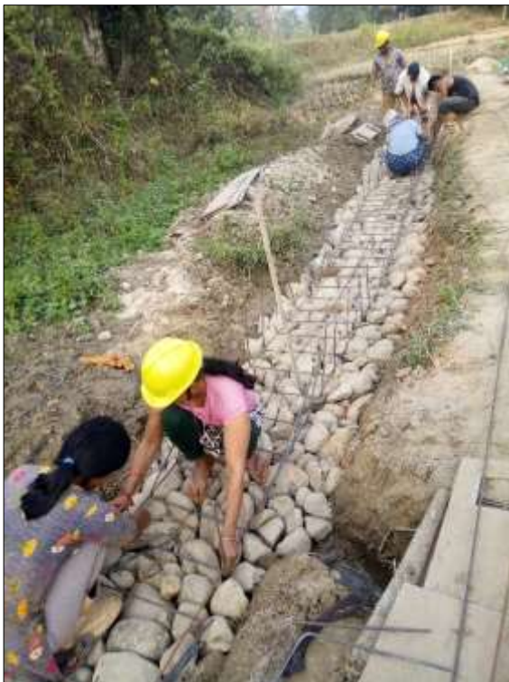
Ms. Shanti Thapa Magar binding the reinforcement bar in Debrepani Irrigation Scheme
