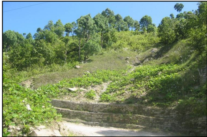
Fig 1: Example of bio-engineering work
