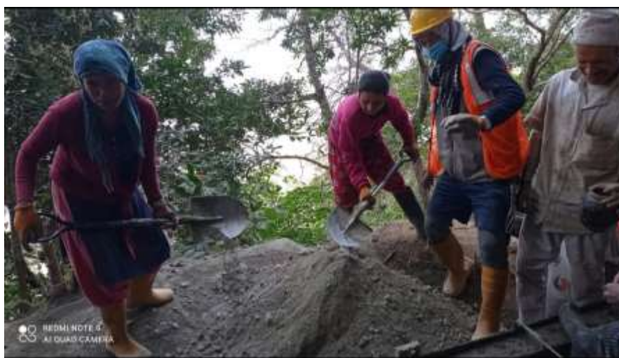
Ms. Gita Bhujel preparing concrete mix for the construction of Simle irrigation canal
